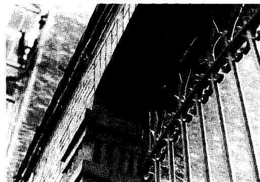
Figure 4 Photograph of a facade hole seen from the outside. The outer face (to the left and up to the gate) is pressed brick, and the inner face is common brick
