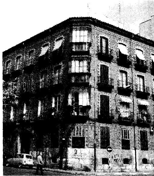
Figure 7 1883 building with ornamental features devised with two-colour bricks placed around the holes and at the strikes with the frame
