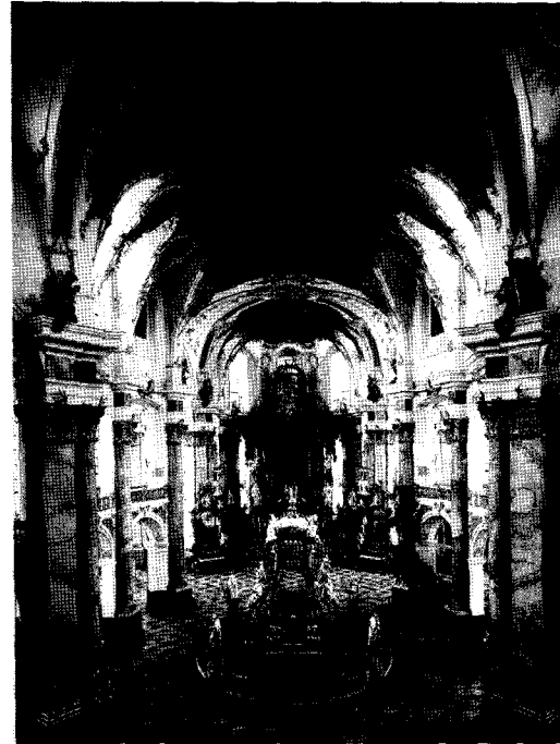
Figure 11 Internal view of the shell
