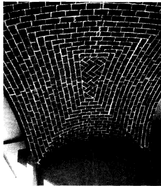
Figure 4 General view of the vault with 4 supporting points
