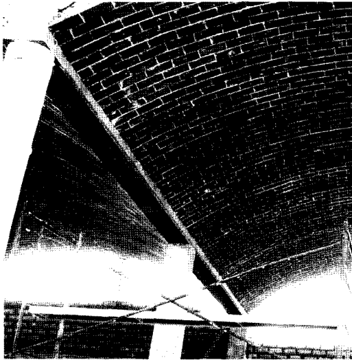
Figure 5 Vault with lineal support over reinforced concrete beam
