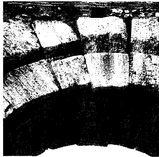
Figure 14 In an arch located towards the Fora, again on the third tier, there is a correction in the groove cut into the face of the arch, made during the course of the works. Obviously there was no reason to make such a correction if this operation was carried out exclusively to aid the adhesion of the concrete and therefore would have remained concealed
